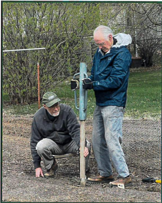
Kent McClelland and Charlie Duke work on placing the posts.
